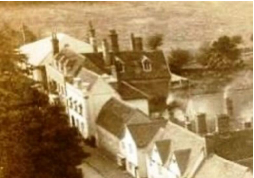
Great House c.1910, still much as it must have appeared in the Wormeleys' time. Note the substantial earlier wing at right angles to the mid-eighteenth century front of the house. The property included a coach house and stable building fronting the High Street and a brewhouse lying behind it (now Littlegarth house and studio).
