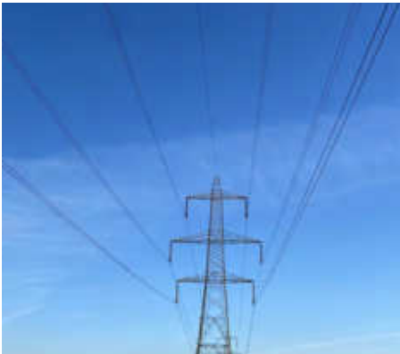
Example of a 400 kV steel lattice angle pylon
